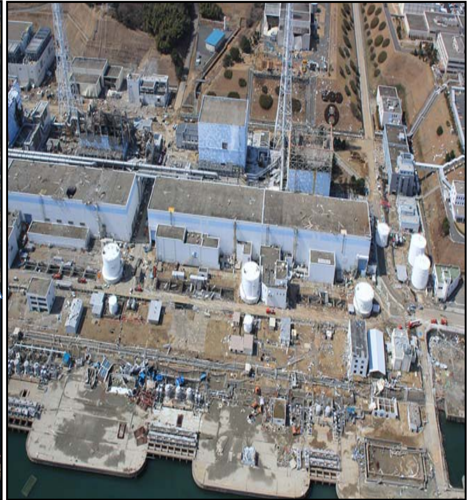
After the Earthquake and Tsunamis
